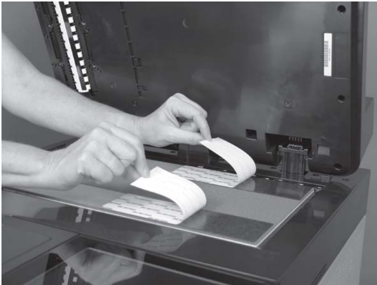
Figure 1-85 Install a replacement document feeder white backing (4 of 9)
